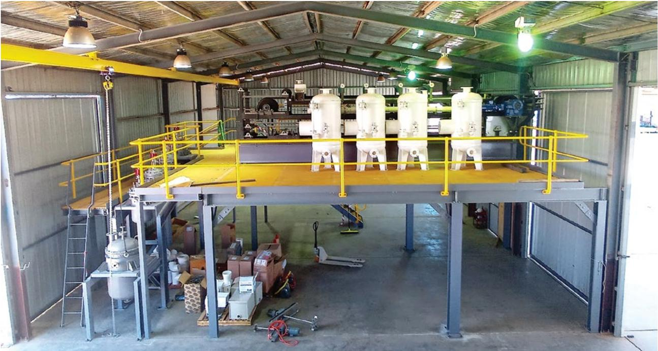
Figure 2 – Pilot Plant Progress – installed autoclave reactors in foreground
